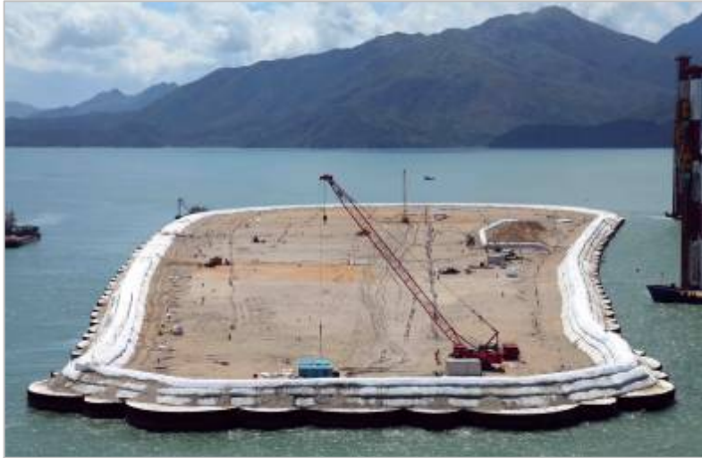
Tunnel Man-made Island (East Island)
