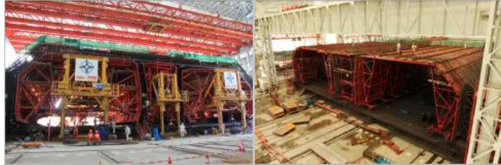
Immersed Tube Tunnel - First segment of tunnel section started casting
